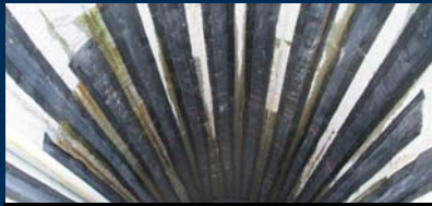
Building the shaft liner - climbing deck not yet installed.
