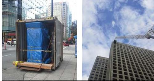
**1075 West Georgia Project: Equipment ready to be unloaded, and later being flown up to the 27th floor by a 475 foot crane.**
