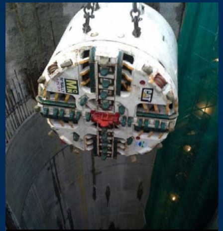
Cutting head is lowered down the shaft - 155 tons on the hook.
