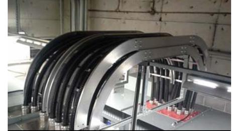
**1075 West Georgia Project: Single conductor cables from the secondary side of one of the transformers to the 600V distribution.**
