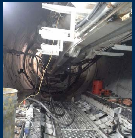
The segments are landed and staged for install under the screw auger.
