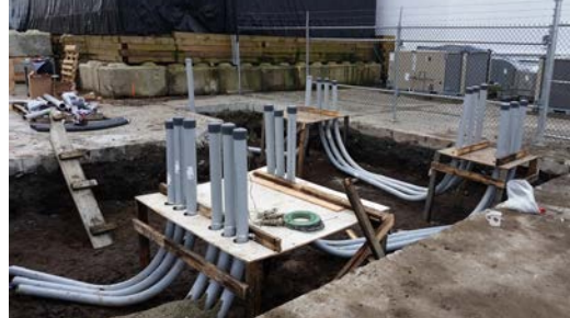
Just behind our old office, Southgate homes "temp" power rough in.
