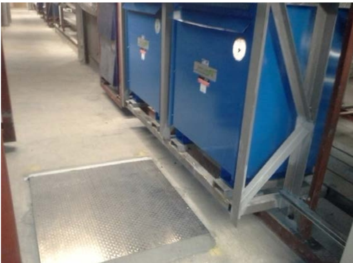
The transformer was raised through the access hatch.
