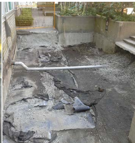
Patio excavation was required before the slab was poured for the generator. Kevin Selesky, Foreman on the project said, "It's a challenging site... we have to work in some very crowded mechanical spaces."
